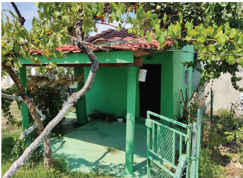
Fig. 12. Exterior view of 'Ali Naime Baba Türbesi'.
