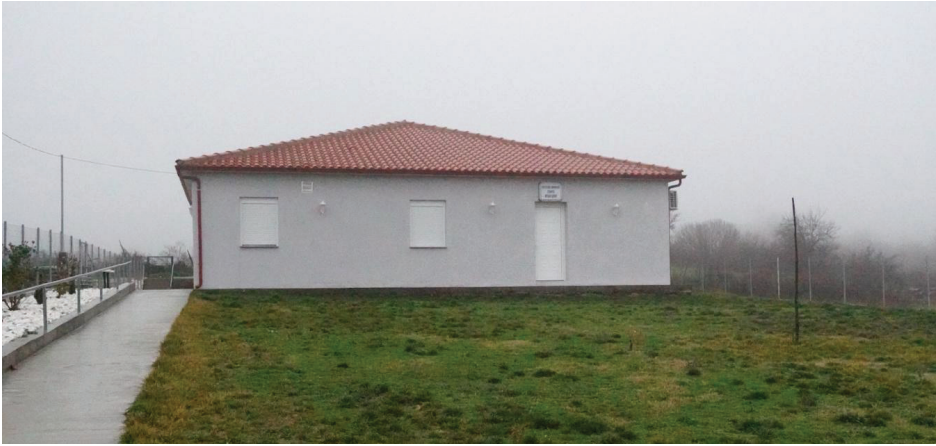
Fig. 6. Exterior view of cemevi in Megalo Dereio (Büyük Derbent).
